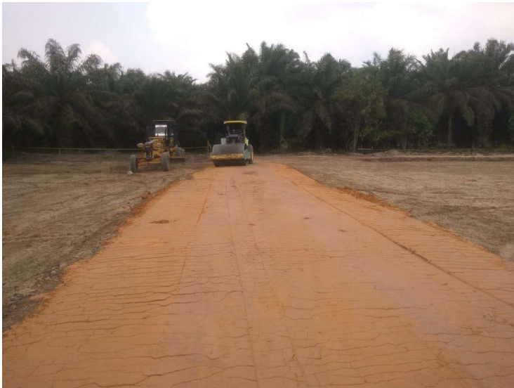
PB-1 Well site construction
