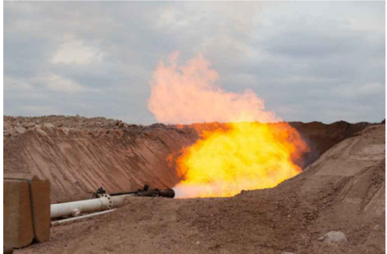
PV-12 Flare during interim flow testing
