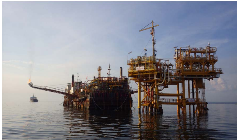
Oyong Well Head platform prior to removal of Oil production facilities and FSO
