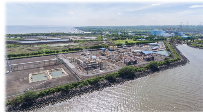
Existing pipeline to shore
